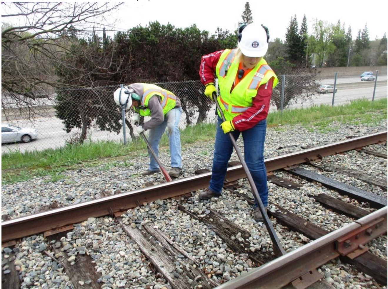
At the job-site, Steve and Bev get right to work pulling spikes the old fashioned way
