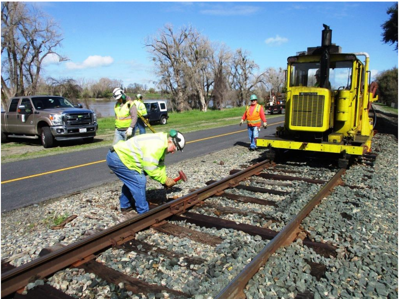
Frank sets spikes on the few ties that didn't get spiked-down last time
