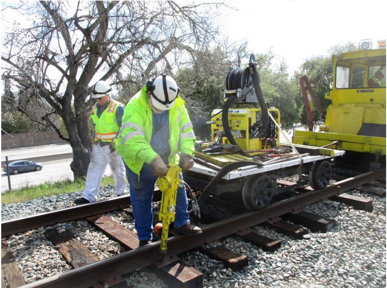
Frank uses the hydraulic spike driver to drive spikes
