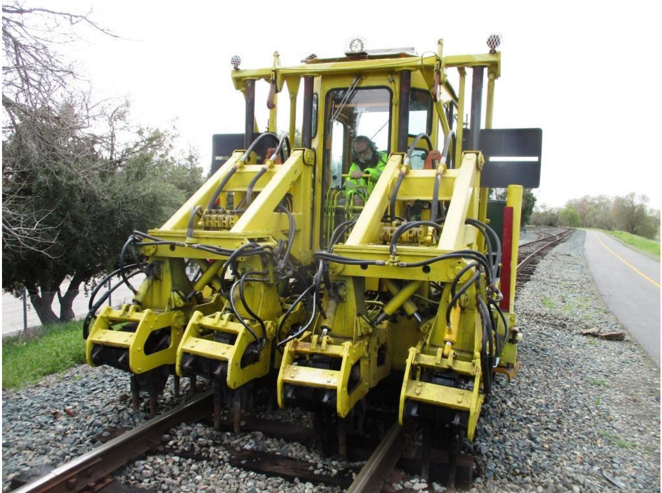
With the tamper now working, Alan tamps the new ties that the Team has installed over the past several weeks
