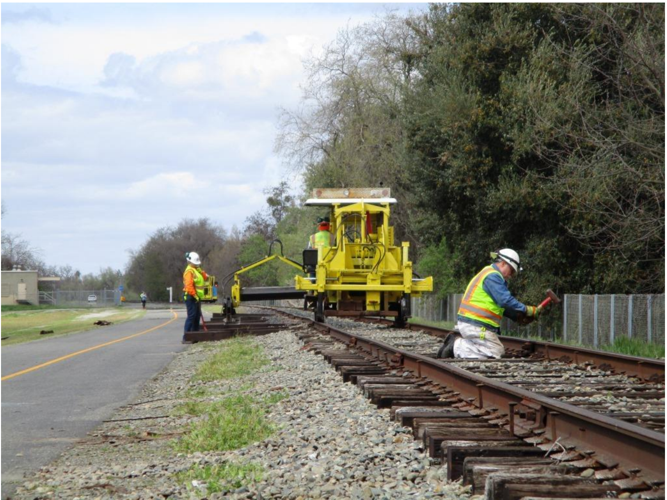
Mike H. sets spikes on all the new ties while Ed and Bev continue pull in more
