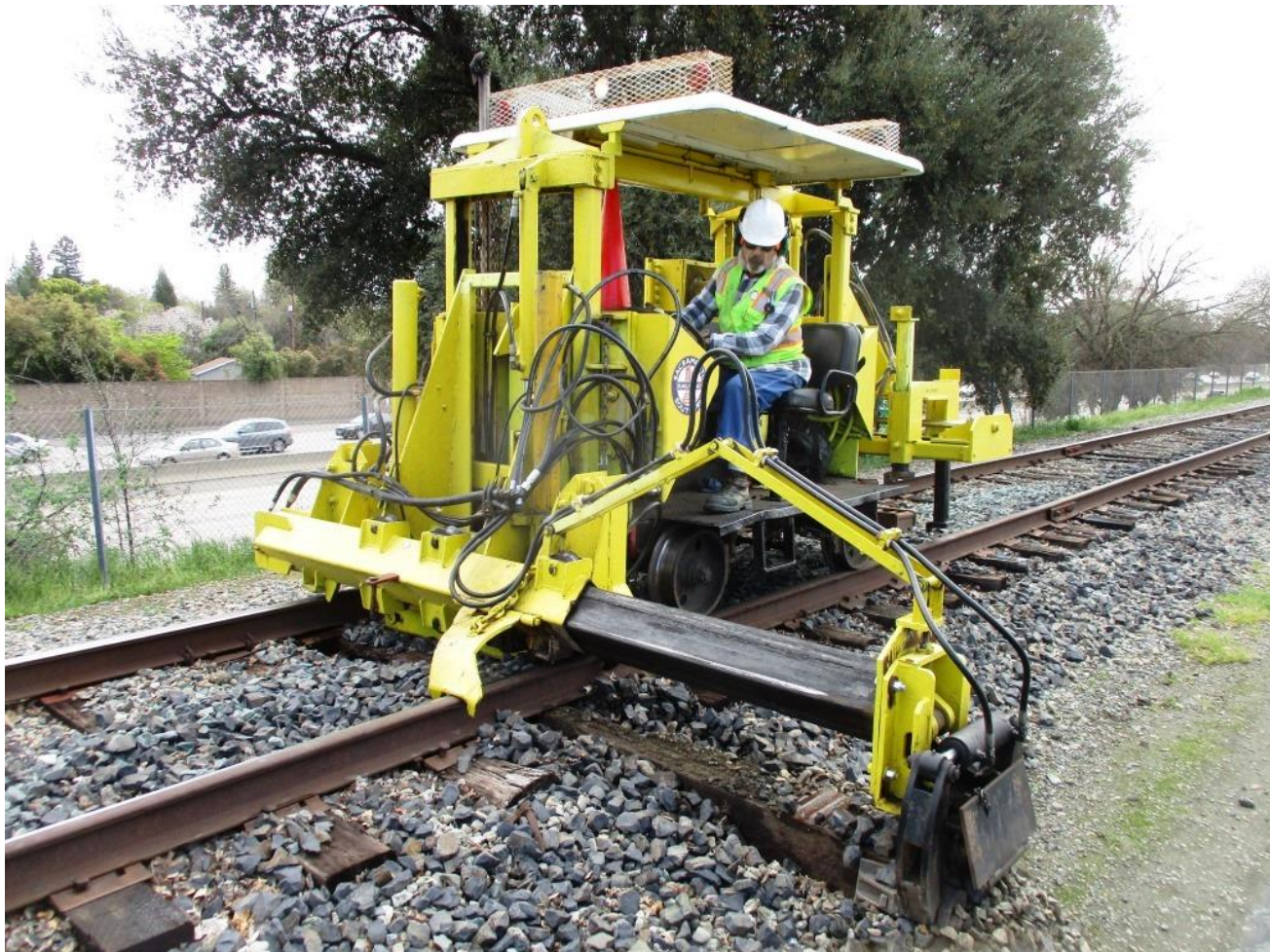
Ed starts pulling out the bad ties with the Jackson 125 tie-exchanger
