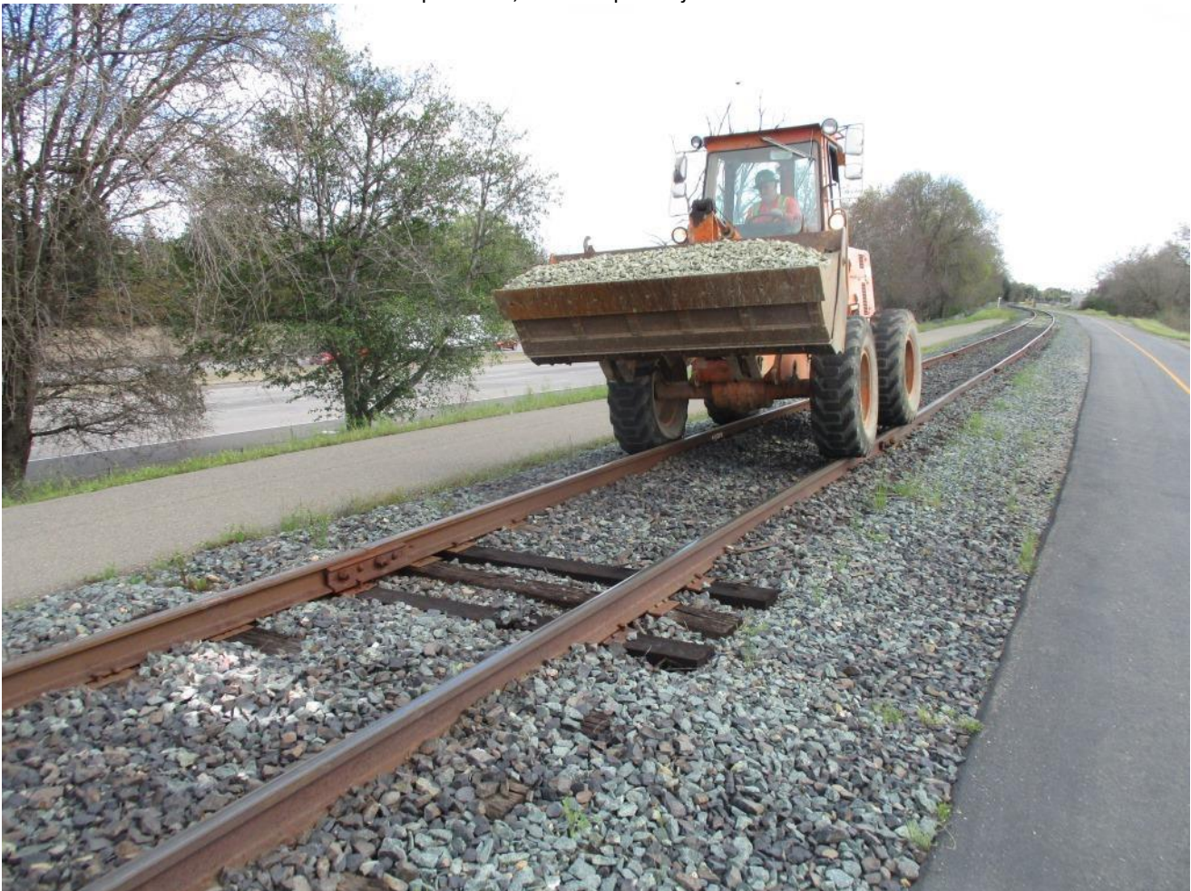
Al in the loader brings a bucket of rock to fill in around joints to provide a better base for the tamper to tamp
