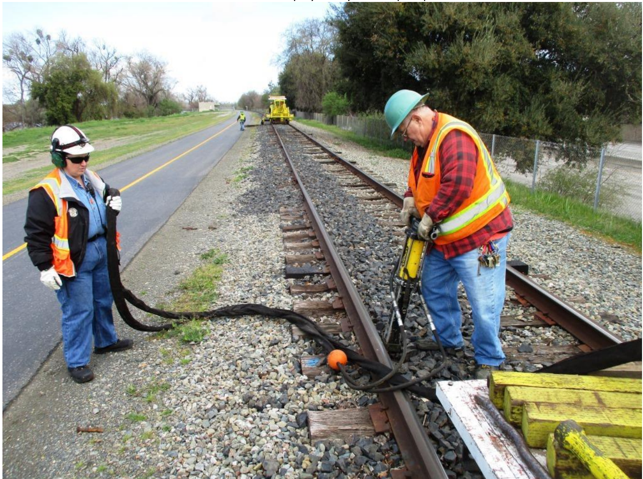
Al takes over pulling spikes with the hydraulic spike-puller
