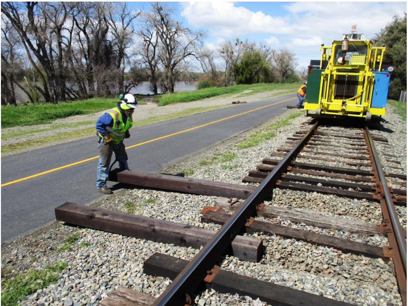
Joe lines new ties up for insertion into the empty cribs
