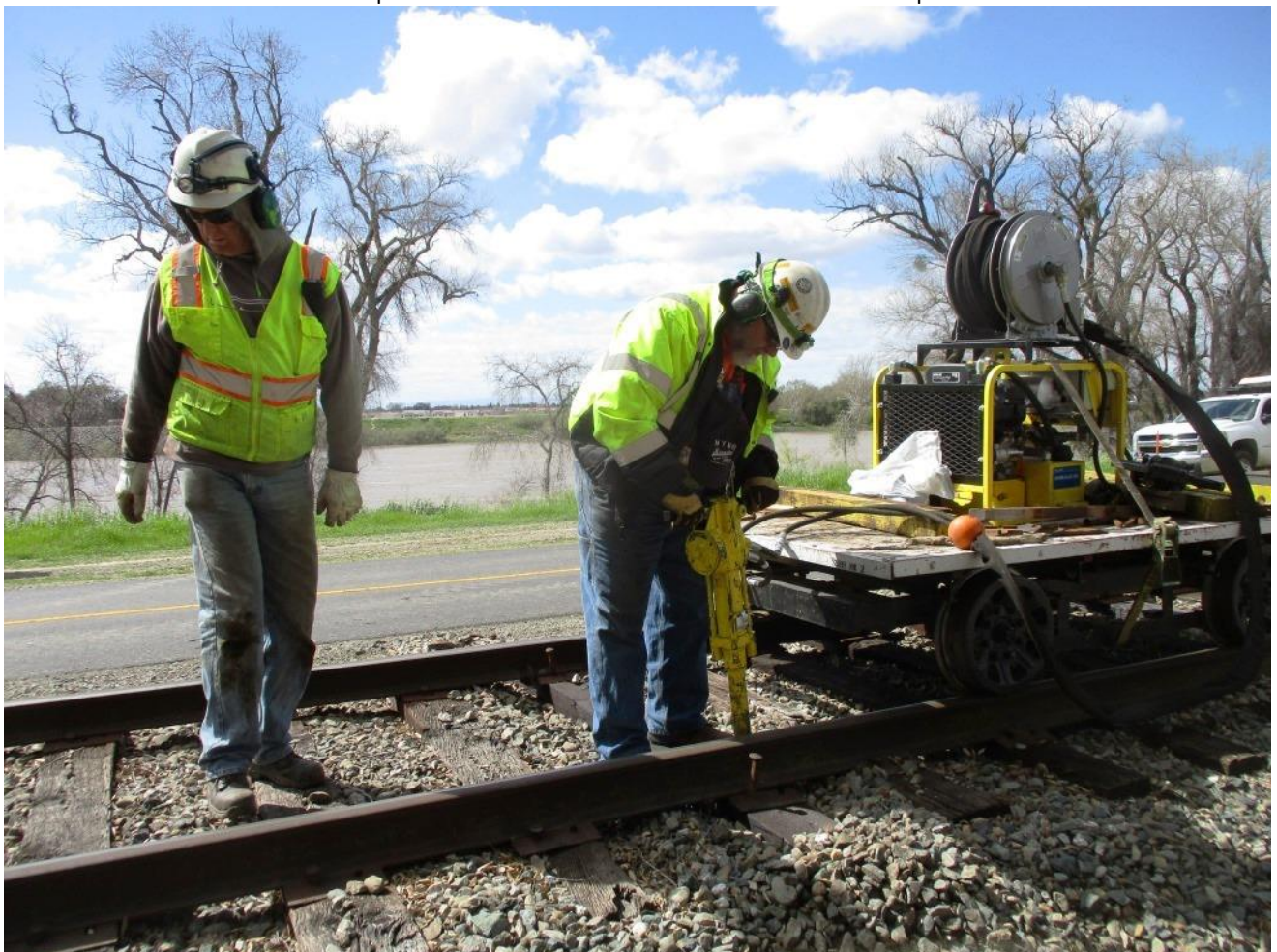
Steve and Mike F. deploy the hydraulic spike-driver
