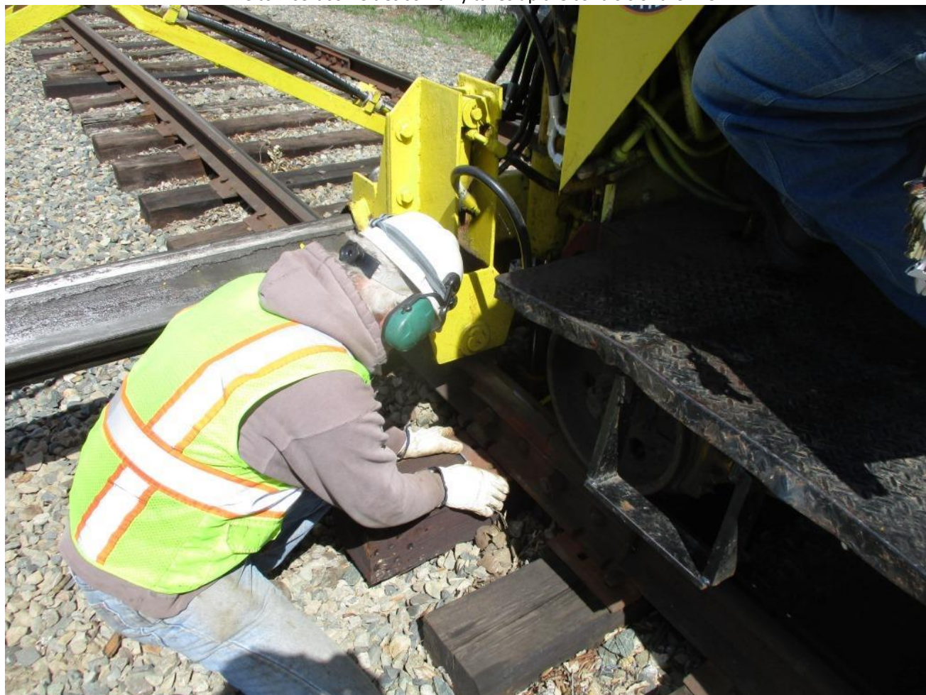
Steve inserts a tie-plate after Harry uses the 125's track-jacks to lift the rail slightly
