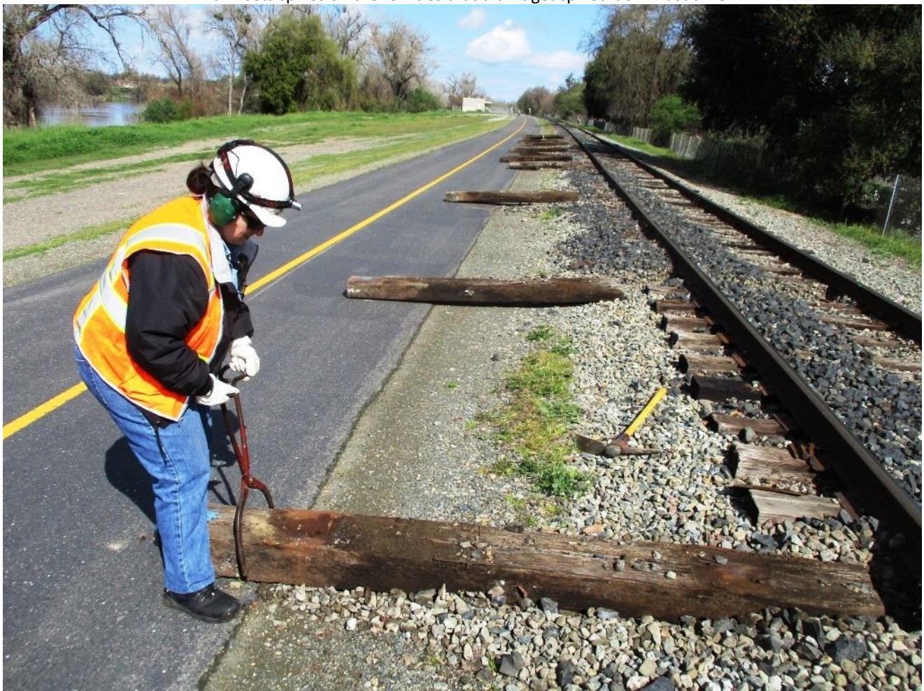
Heather moves a dead-tie out of the way so that GM2 can scoop it up
