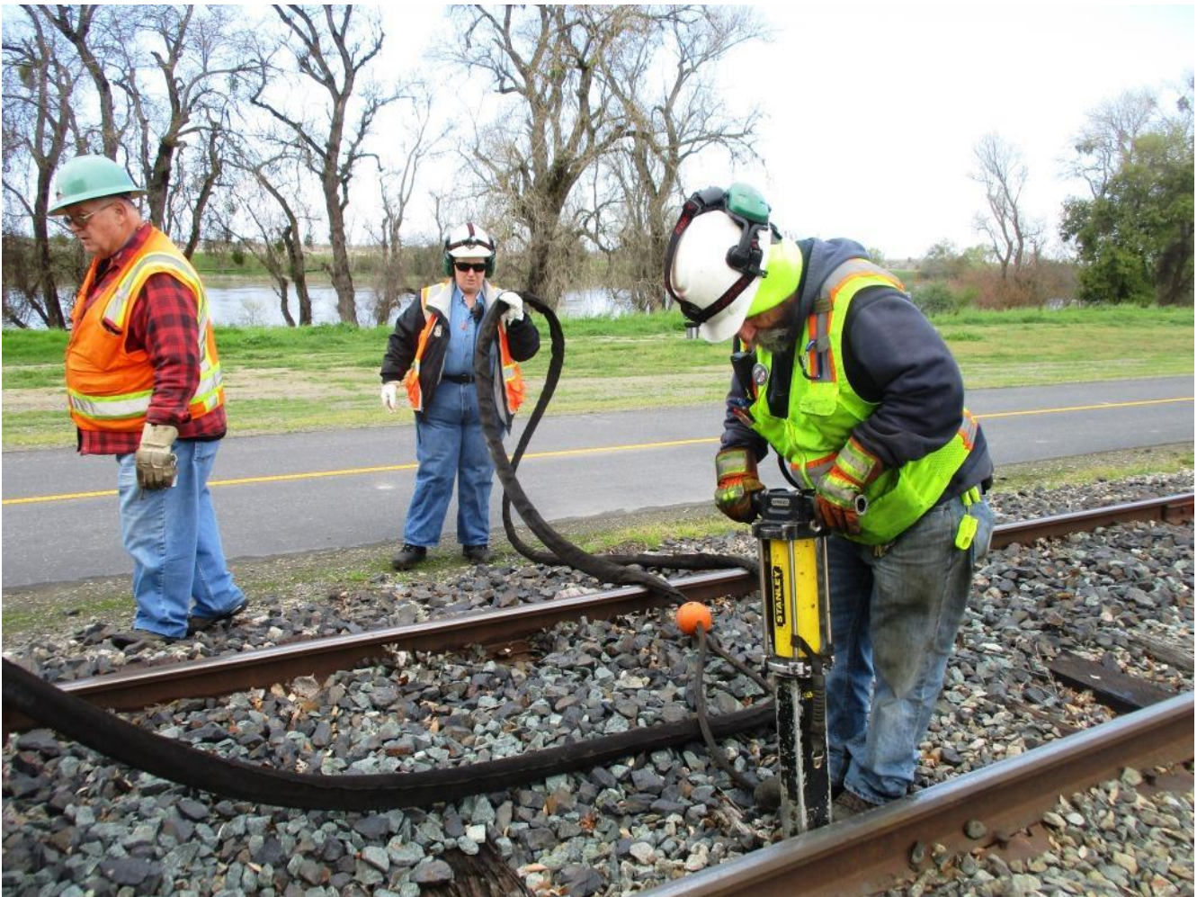
Joe and Heather deploy the hydraulic spike-puller
